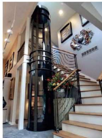
A vacuum-operated home elevator installed by Arrow Lift. CREDIT: ARROW LIFT
